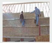
L. The subroof or roof sheathing is applied from the bottom up with temporary traction boards nailed to the subroof to allow safe installation of the material.
