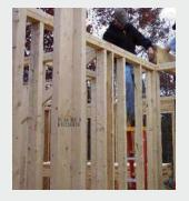
The interior wall framing is composed of studs traditionally referred to as 2×4s. The horizontal member at the top of the studs is called a girt or a ribbon. In this case the builders have used two 2×4s, placing one on top of the other. Because the outside walls
