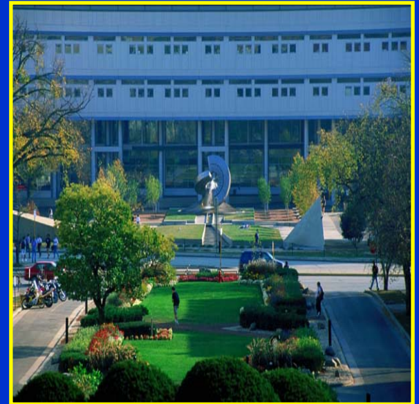
Engineering Hall, University of Wisconsin, Madison, USA
