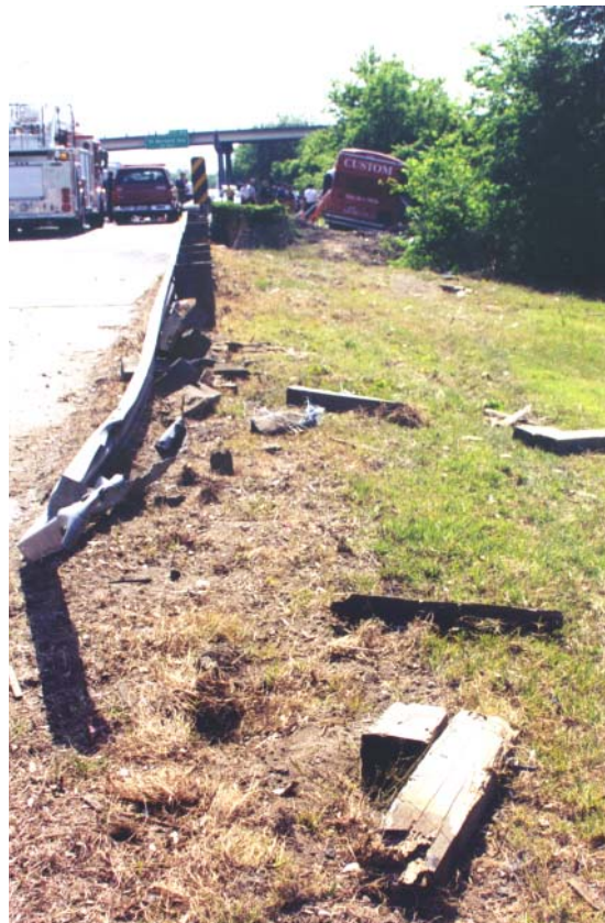
Figure 4. Fractured wooden posts at accident site.
