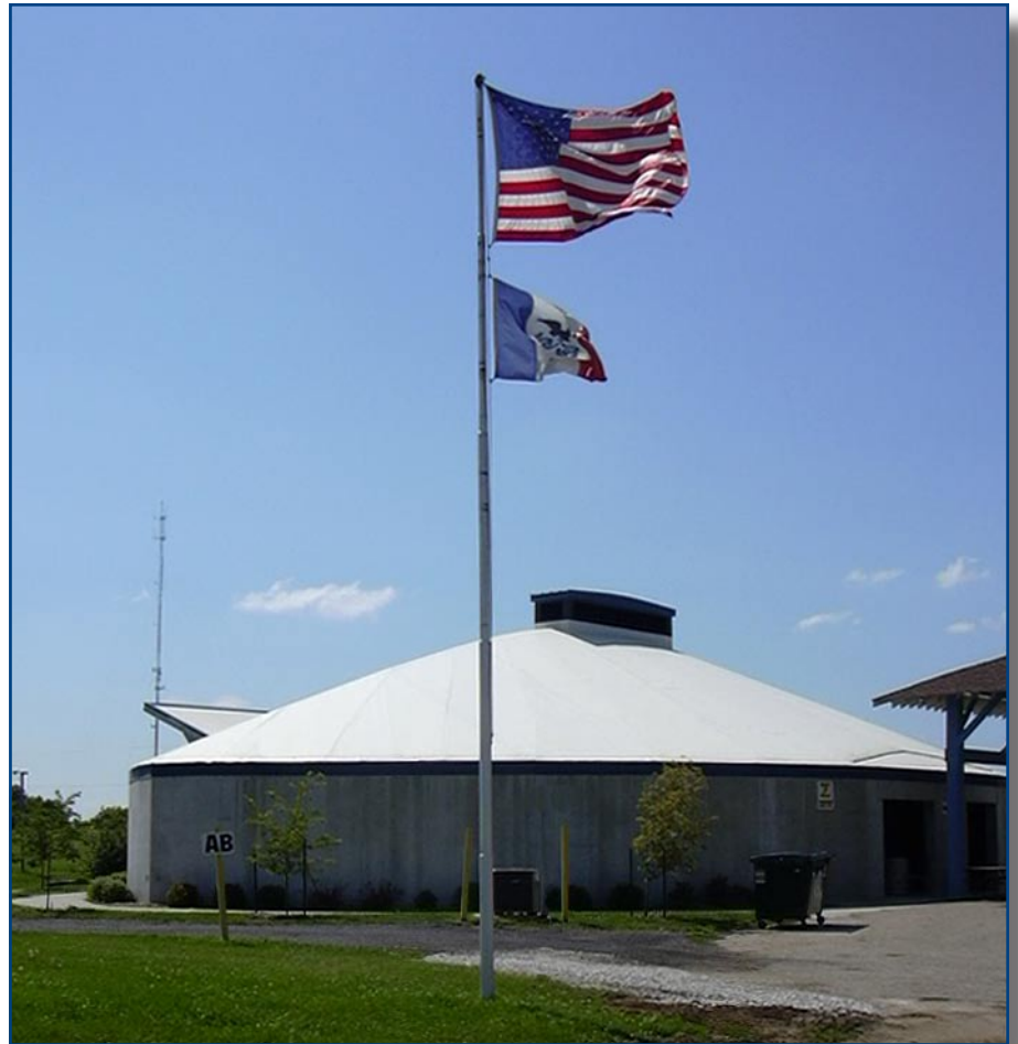
Completed shelter. SPATIAL DESIGNS ARCHITECTS AND CONSULTANTS
