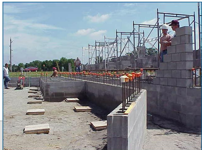
Construction of fully reinforced CMU interior partition walls.
