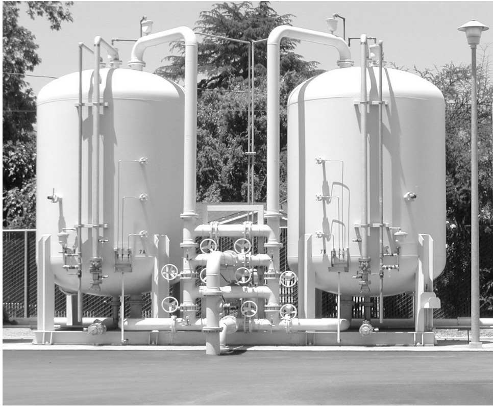
Photo 34. Typical Carbon Vessel Pair (Subsection 4.3.1.1)
