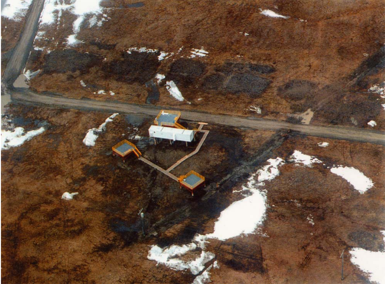
Figure 5.8. Aerial View of PAARCS and Instrument Platforms (W/O Instrumentation)
