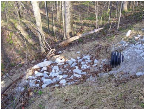
A culvert outfall protection on an oil and gas road in Little Sandy Creek
