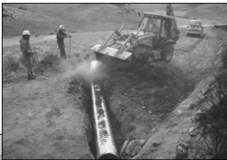
Above, an NPS crew installs a culvert drainage pipe along a road at City of Rocks National Reserve as part of an inter park cooperative project. At left, NPS crews that worked on the City of Rocks road rebuilding project gather for a group photo. Their efforts saved $100,000 in costs for road and parking area improvements at the park in southern Idaho. NPS photos by Wallace Keck
