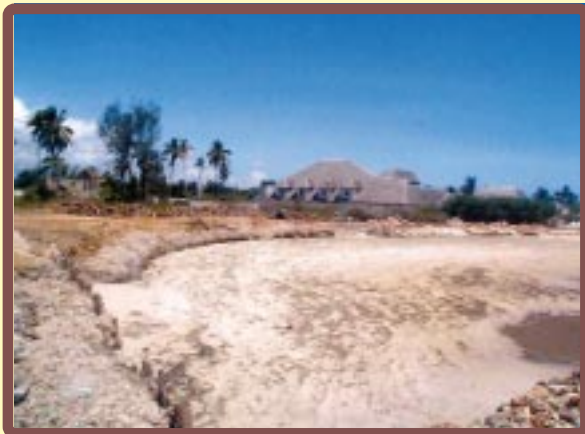
Fig. 2: Most of the erosion around Dar is caused by the extraction of sand for construction and the removal of vegetation in order to develop the shoreline.
