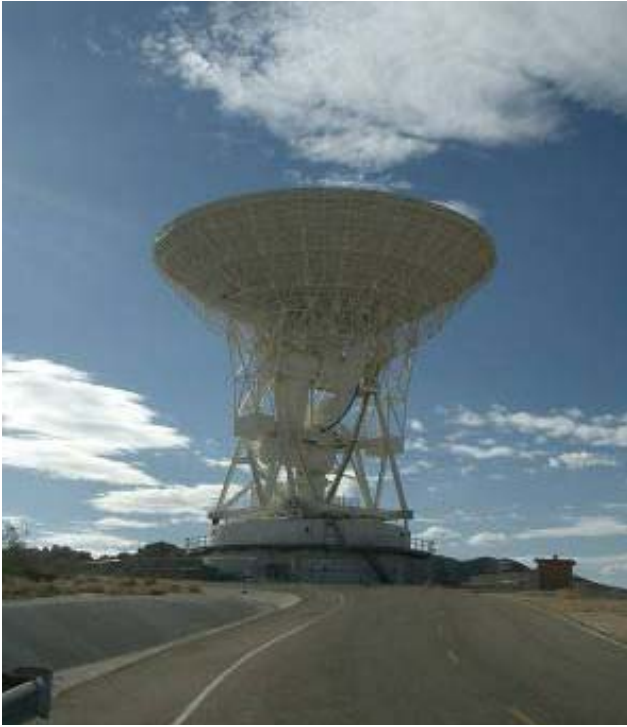
Figure 1 – Photographs of the DSS27 antenna which is identical to the DSS28 which will be modified for the wide band operation described in this paper. The original antenna has a beam-waveguide optical system which guides the beam through the 2.74m diameter hole at the vertex, through mirrors, to a large stationary control room in the antenna base. The revised system will utilize a tertiary reflector covering hole with receivers located near the vertex.
