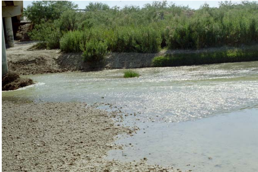
Photo 7: Rio Grande at the International Bridge
