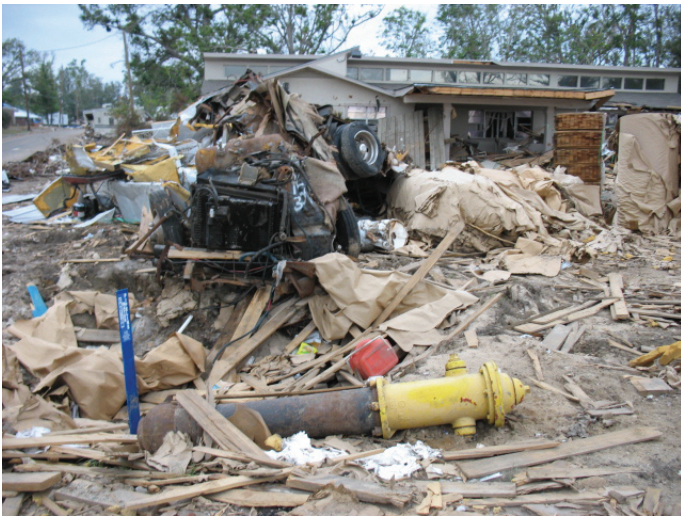
Destruction in the wake of Hurricane Katrina
