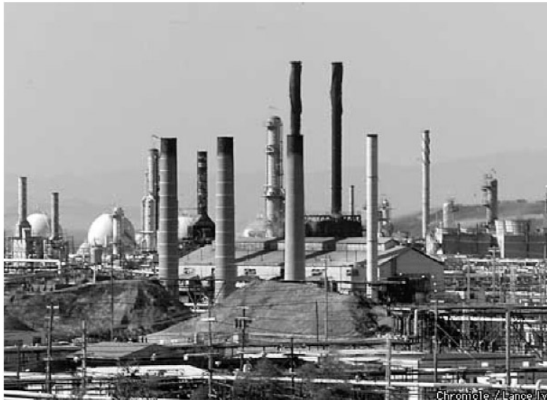
Figure 11: General Chemical Facility Co-located on Chevron Richmond Refinery Property
