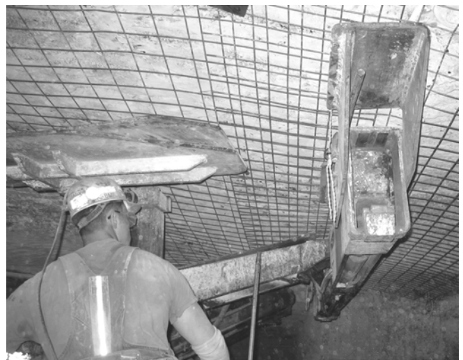
Figure 2. Screen providing protection during bolt installation.
