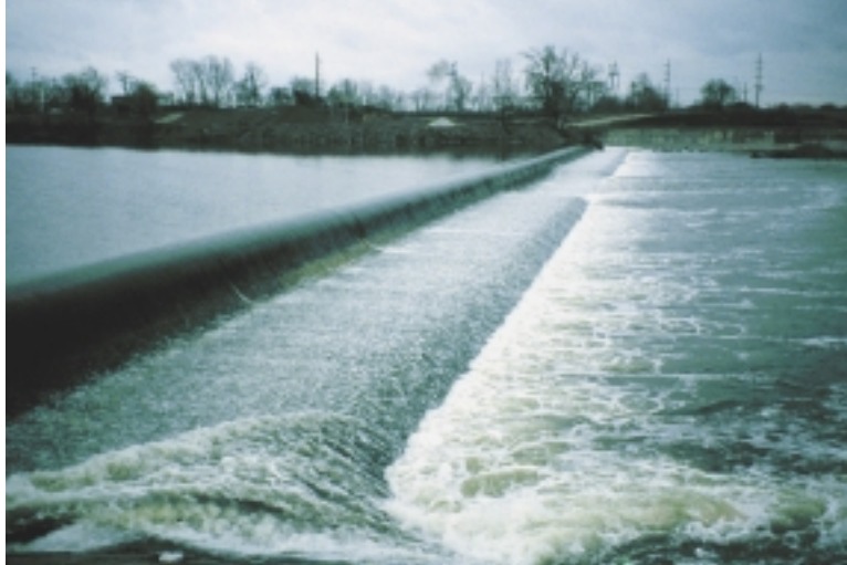
Figure 3-2. A low-head dam can be a hazard during a field effort. They are particularly hazardous because they are difficult to see from the water.
