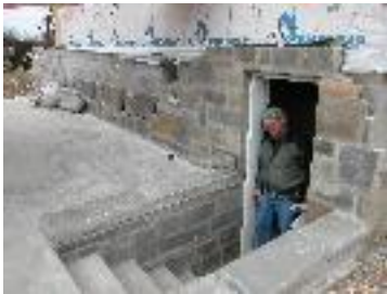
Donnie Fletcher standing in doorway of the subterranean storm shelter which was completed three weeks prior to the EF4 tornado.
