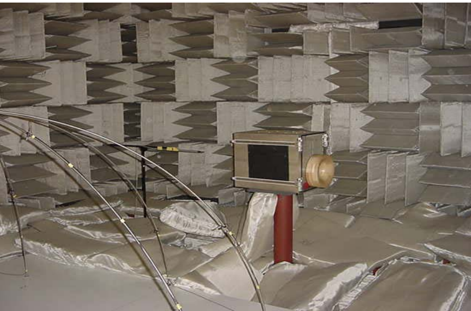
Anechoic chamber with habitat on pedestal. Sound power reflection plane and hemispherical microphone grid to left.
