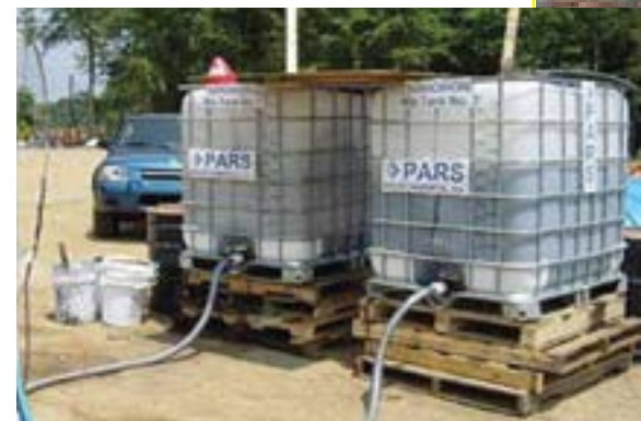
An injection setup for nanoiron slurry.
