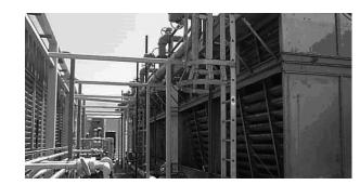
Figure 1 Cooling Towers from a Chilled Water Cooling Plant
