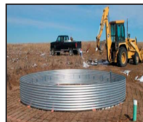
A stock tank being installed on the Bohart Ranch.
