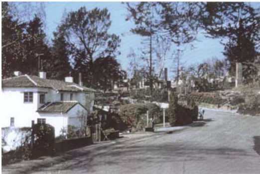
Figure 1a. Spotty damage to homes and vegetation at the periphery of the 1991 Oakland Hills fire area.
