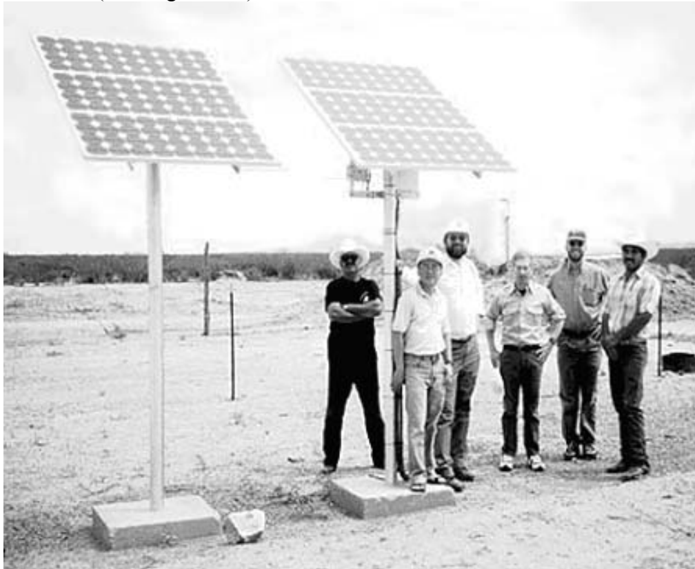
Figure 1. A photovoltaic water pumping system at Colonia Modelo, Chihuahua has improved overall ranch profitability since it was installed in March 1997. After that time, three other photovoltaic water pumping systems have been installed in the area.
