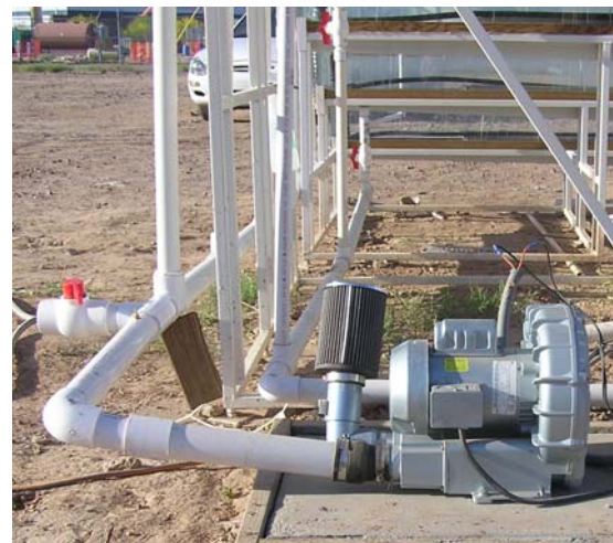
Figure 6. A Sweetwater regenerative blower for culture aeration.
