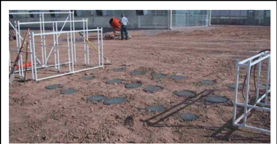
Figure 3. Nine small concrete pads to support the steel frame.
