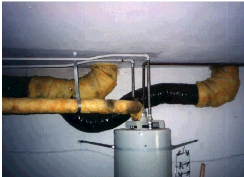
Figure 5. Combination of plastic insulated flexible duct and added open face glass fiber insulation
