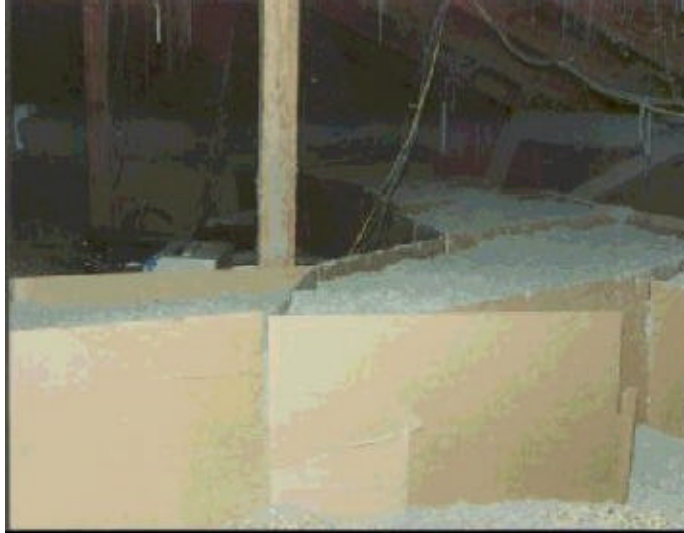
Figure 6. Blown in place duct insulation
