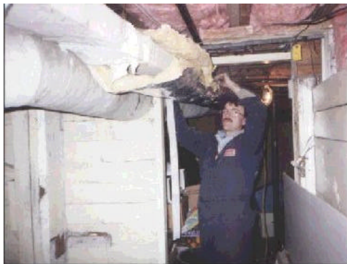
Figure 7. Installing extra duct insulation
