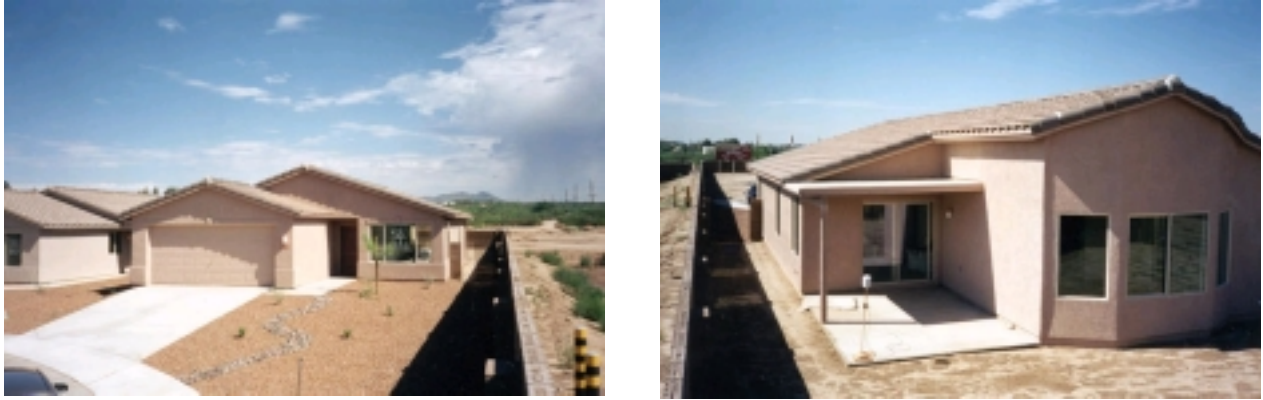
Figure 25. Front and rear views of Tucson prototype house
