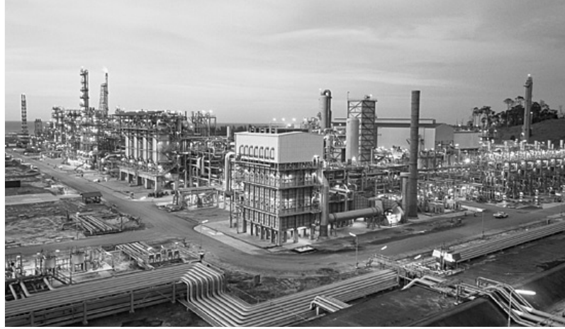
Courtesy: Royal Dutch Shell's Bintulu SMDS facility
