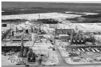
Phase 1 under construction, Jan 2006, Source: OPTI Canada Inc.
