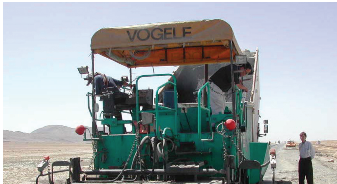
USAID-supported subcontractor paving a section of Kabul-Kandahar highway in August 2003.
