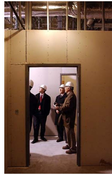
Robert DeGezelle (right), project manager at the new St. James Health Health Services facility, explains building features to Steve Wenzel (center), state director of the USDA's Rural Development, and Andy Burmeister, constituent policy liason for Sen. Norm Coleman, Thursday during a tour of the site.
