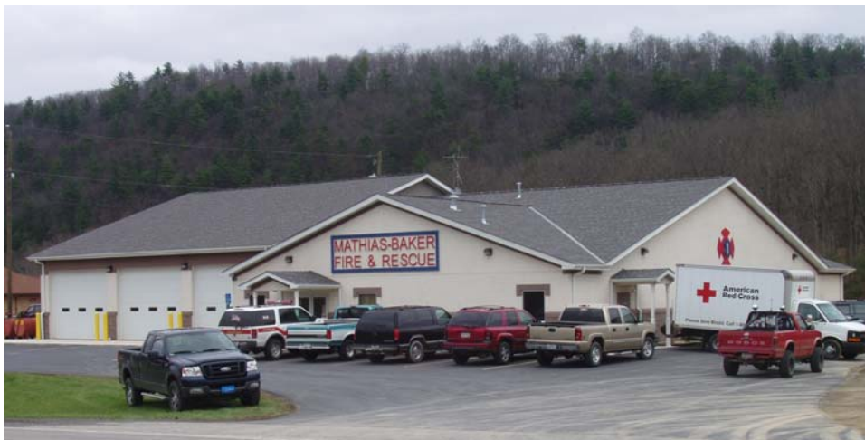
The Mathias-Baker Volunteer Emergency Squad, Inc. new facility in Baker (Hardy County), WV.
