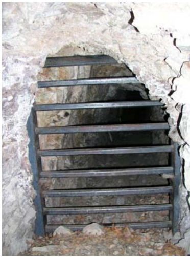
Bat gate, State of Texas mine, CNM
