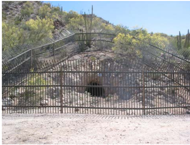
Bat fence, Blue Bird mine, Cabeza Prieta NWR
