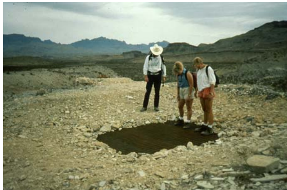
Grate steel mesh covering, Courtesy: John Burghardt
