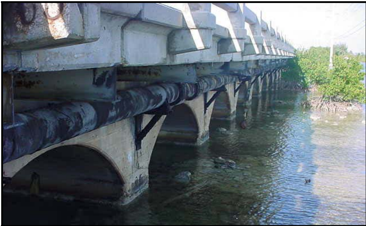
Plate 4: Old Bridge Showing the Construction Techniques and Force Main, Alternative 2.
