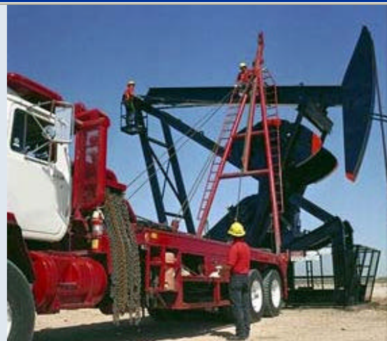
Fig. 2. Servicing horsehead and bridle
