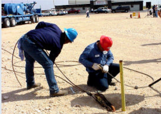
Fig. 6. Installing guy line anchor
