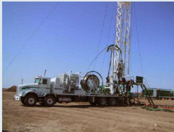
Fig. 22. Installing coil tubing
