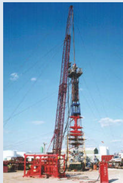
Fig. 21. Snubbing rig with blow out preventer (BOP)
