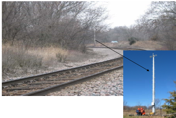
Figure 3. Access Point Antenna Pole on the Farther Side of Curve
