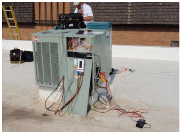
AirCare Plus contractor (in background) servicing a packaged rooftop unit.
