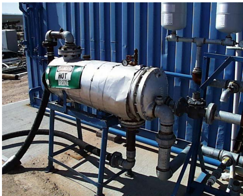
Figure 13.—Intermediate heat exchanger.
