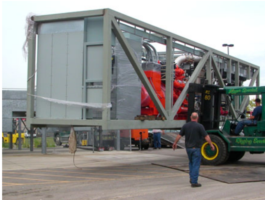
Figure 9: Offloading of Cogeneration Module
