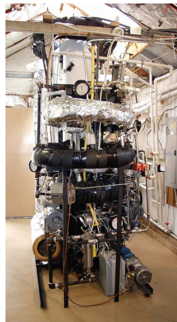
Laboratory test model of a Hi-Cool natural gas cooling system.
