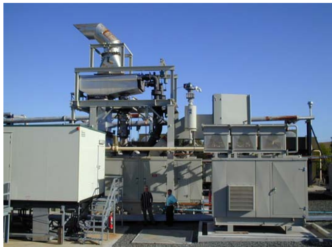
Figure 7. EDL Carbureted Gas Turbine Installation
