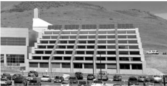
The performance of this 6-kW ac PV array on the east wing of NREL’s Solar Energy Research Facility was compared to an identical array on the west wing (see van Dyk et al.).
