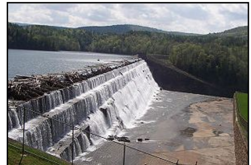
Typical Gilboa Operations before Stabilization
