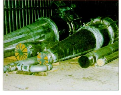
the inner portion of a coaxial pipe and past the hot gas intercept valves on its way to the gas turbine. The cyclones and gas collecting pipe are insulated to minimize gas temperature loss.
