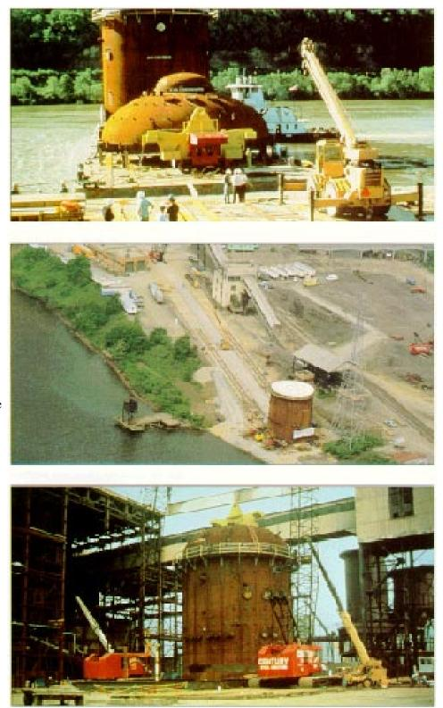
With the barge docked at Tidd, the crew gets ready to oft-load the head, detached for clearance under bridges (top). The vessel shell was moved up a 900-foot haul road, over a steel plate track laid on timber mats (center). With major internal components installed and the head repositioned, the pressure vessel is ready for the final move into the building (bottom). Once in position, the head will be arc welded in place.
