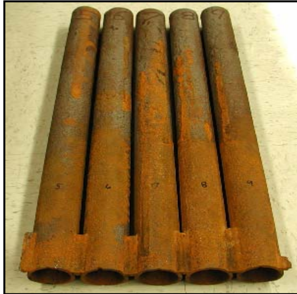
Figure 9. A panel of tangent tubes with suspected stress-assisted corrosion was tested with guided waves.
