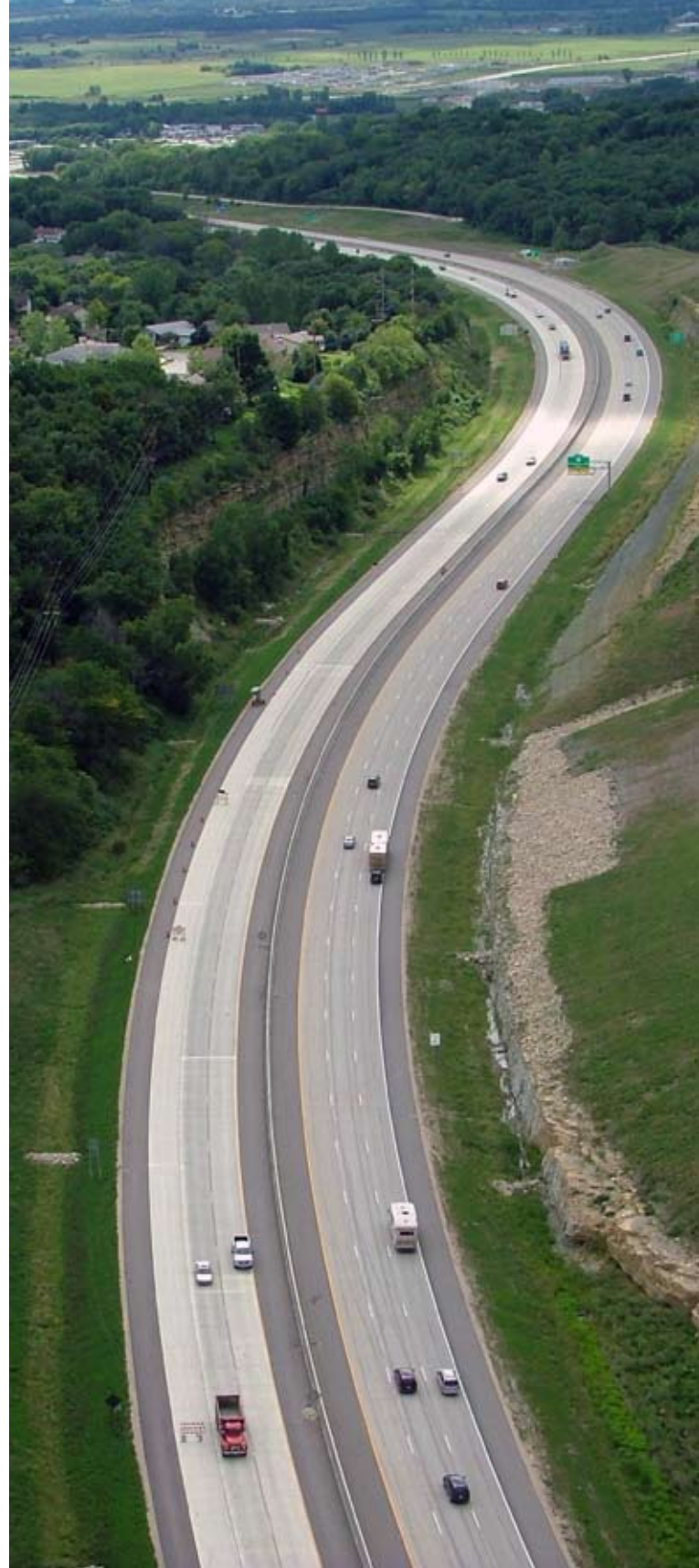
ZRC focused on a 60-year pavement life cycle, using high-performance concrete to reduce long-term maintenance costs.
