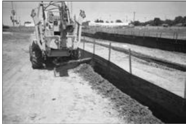
Straight line efficiency testing for trenched and sliced silt fence.
