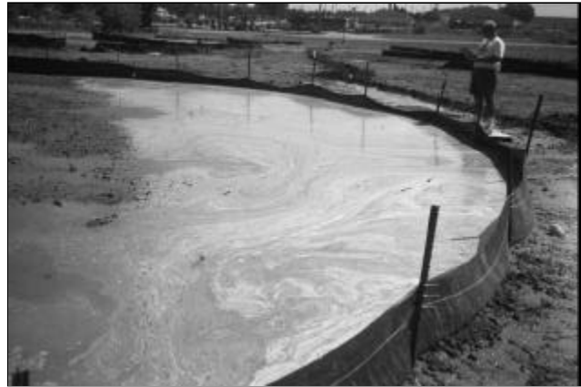
30-foot radius water retention test for slicing installation.
