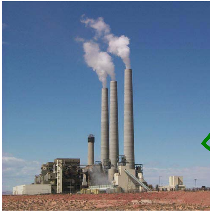
Navajo Power Plant (4 corners NM)
