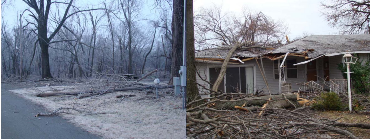
Ice Storm Damage in Cherokee County Kansas
