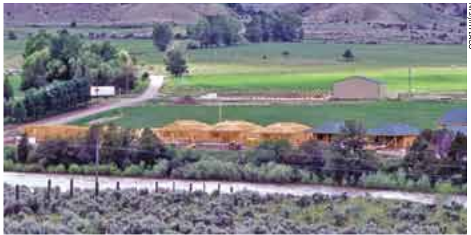
Construction along the Yellowstone River north of Yellowstone National Park.
