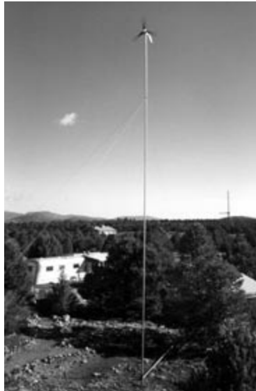
A Southwest Windpower Air 303, 300-watt turbine is the sole source of electricity for this remote home in northern Arizona.
