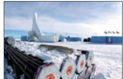
Drill rods await use just outside the ANDRILL building complex.
