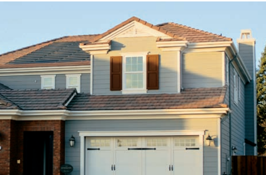
The PV system on this home in Danville, California, consists of 48 BP Solar EnergyTile modules that comprise a 3.1-kW system. This home is part of the Ponderosa community. Credit: BP
