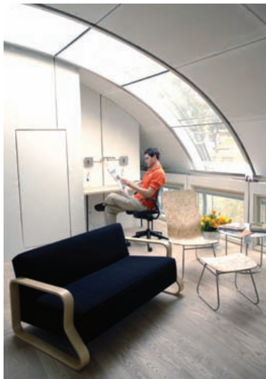
An expansive window follows the roofline of the University of Michigan's 2005 Solar Decathlon house and allows natural daylighting into the work and living spaces. Credit: Chris Gunn, NREL PIX/14268
