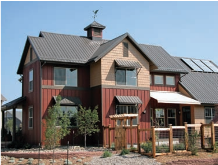
This house, built by McStain Enterprises under the DOE Building America program, contains value-engineered floors, better insulation, tighter ducts, low-emissivity windows, and controlled ventilation to improve indoor air quality. It also features a solar space-heating and water-heating system. Credit: Nancy Wells, NREL/PIX 13551
