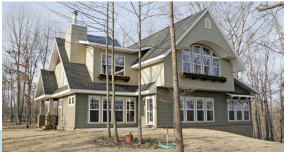
Built by Stitt Energy Systems of Rogers, Arkansas, winner of 15 EnergyValue Housing Awards, this home demonstrates the builder's unwavering passion for energy conservation and use of solar energy technology. It is the 2006 EnergyValue Housing Award gold winner in the Custom Home, Moderate Climate category. This home was also chosen as NAHB's 2007 Green Building Project of the Year. Credit: NAHB Research Center.
