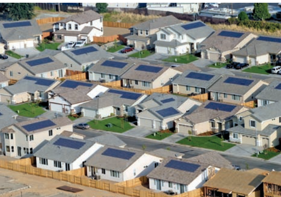
Premier Gardens, a highly energy-efficient community in Sacramento, California, generates more than 50% of its own electricity using GE Brilliance Roof Integrated Solar Electric Systems. Credit: GE
